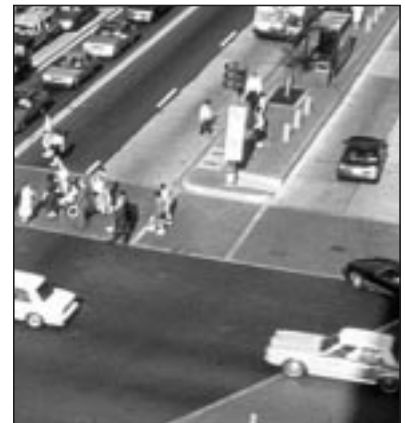
Striping is designed to give the motorist and the pedestrian clear visual cues as to where he or she belongs.
